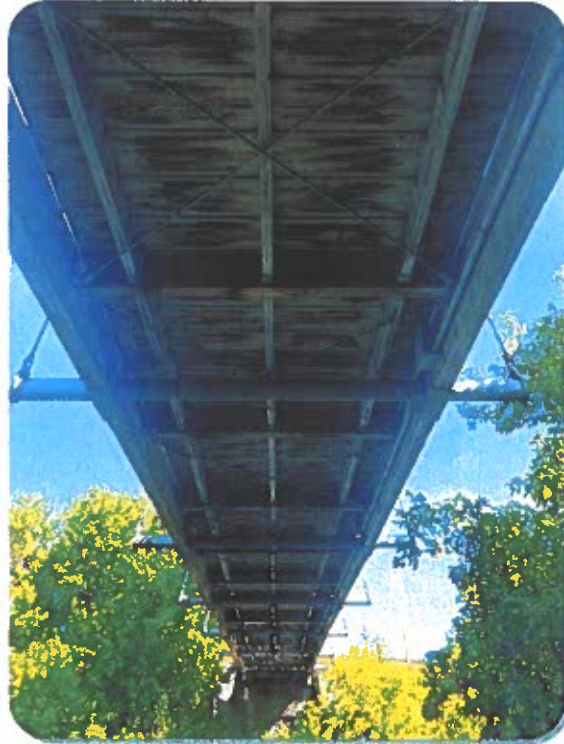
Photo 6: Floor system configuration.
