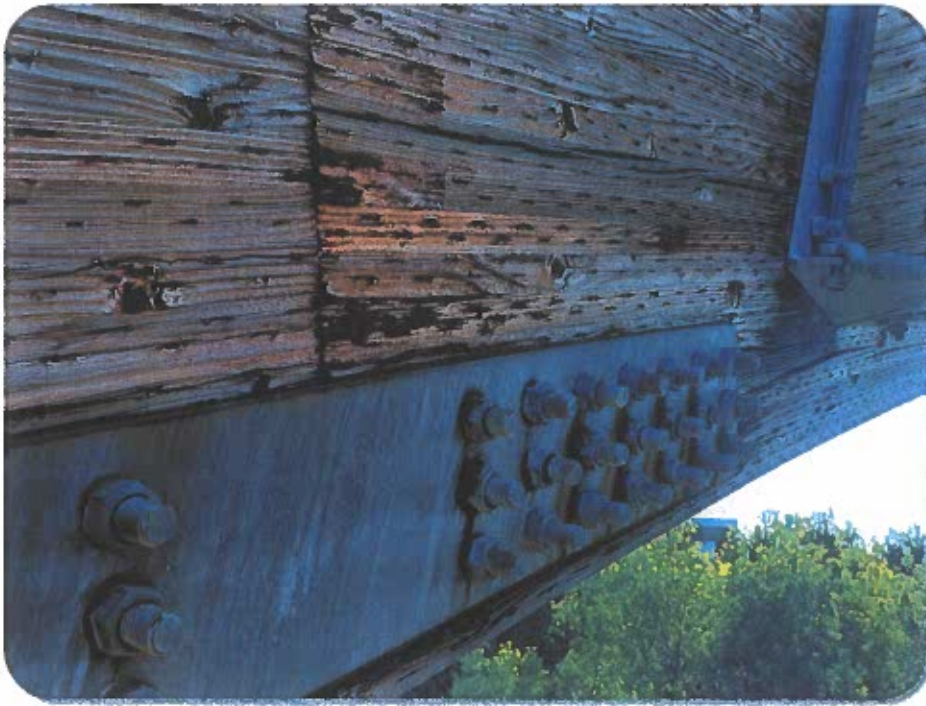
Photo 3: One-third point splice
