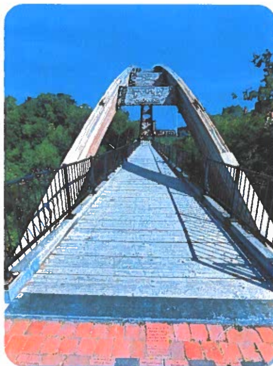
Photo 14: West approach slide plate.
