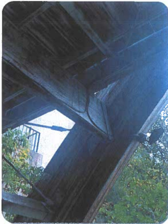
Photo 11: East transverse strut.
