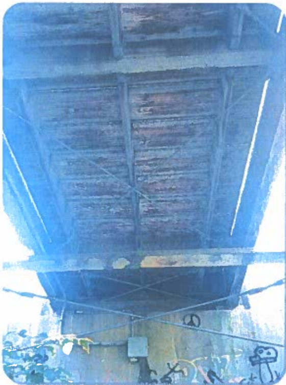
Photo 8: Floor system diagonal tension rods.
