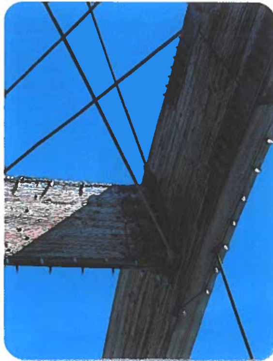
Photo 5: Arch diagonal tension rods and cross braces.
