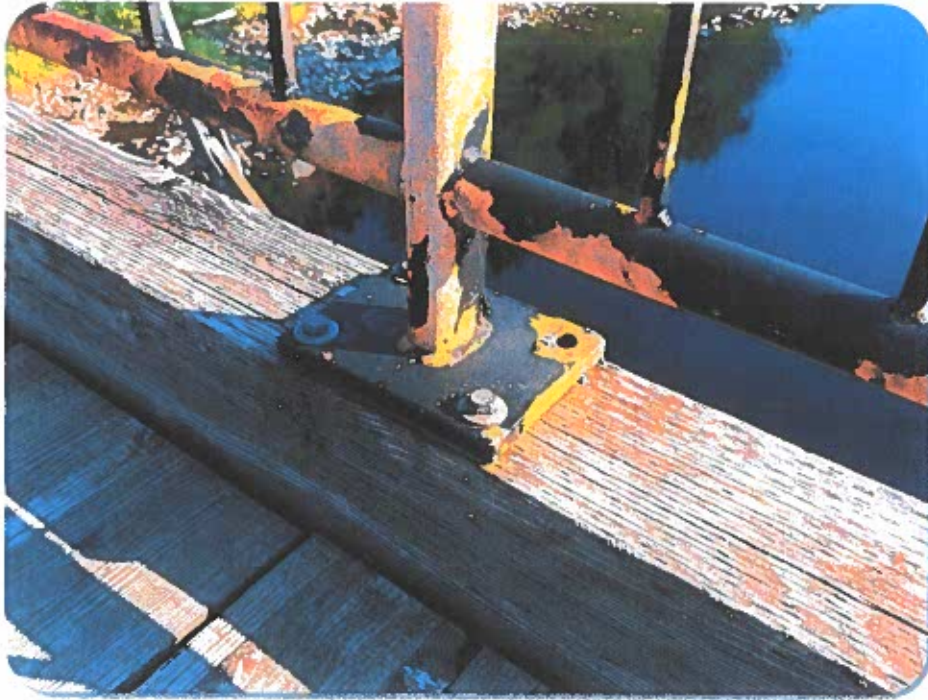
Photo 9: Rail post base plate.
