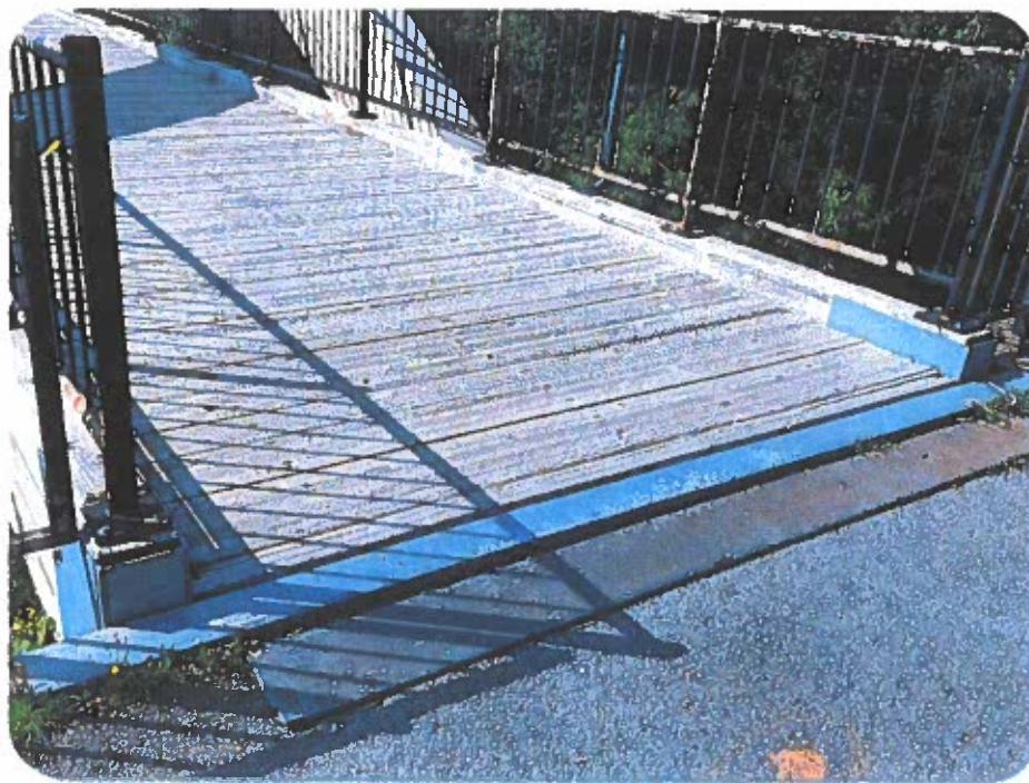
Photo 13: East approach slide plate.
