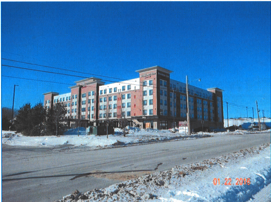
Looking easterly from Bass Park Blvd. REQ
