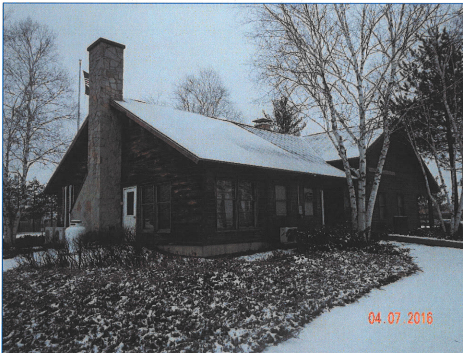
Looking northwesterly at improvements REQ
