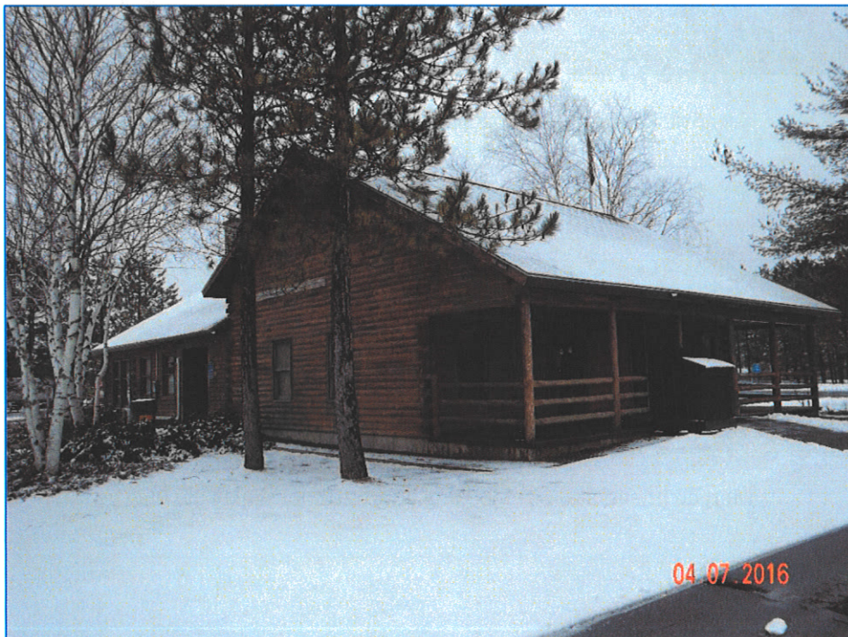
Looking Southwesterly at improvements. REQ
